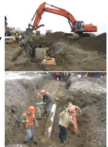
East Front Street Construction
