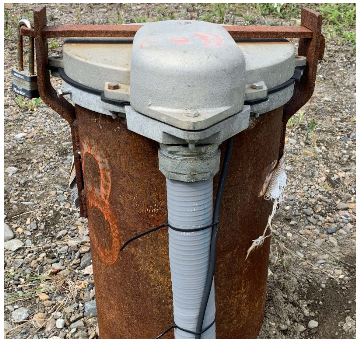
Well #3 – Conduit & well cap secured on June 27, 2019
