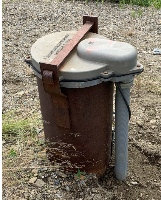
Well #2 – Conduit secured on June 27, 2019
